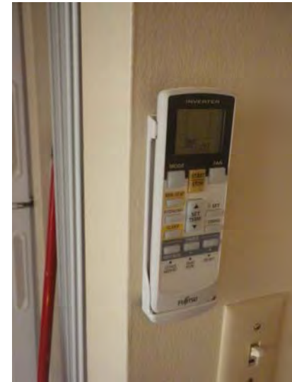
Heat pump controls
