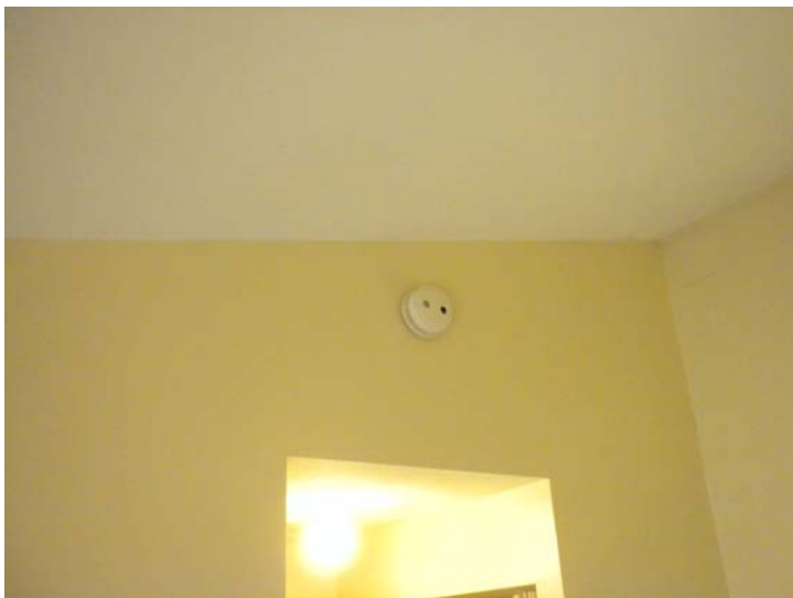
Hardwired smoke detector
