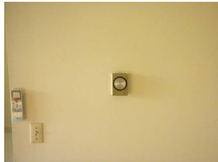
Original thermostat controls for electric baseboard
